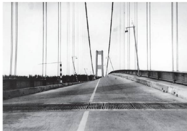
Figure 13.22 The Tacoma Narrows bridge disaster
