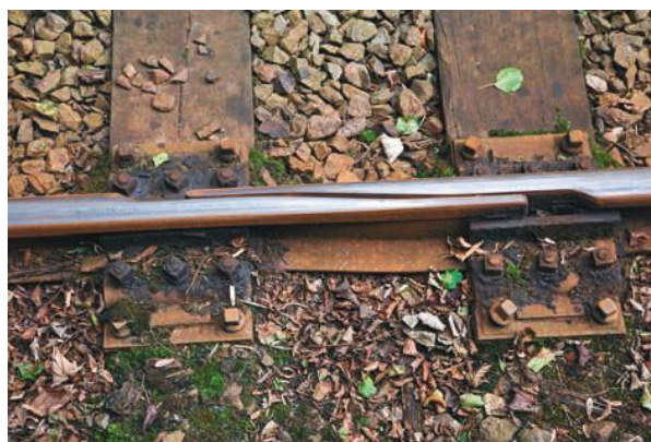
Figure 19.2a Tapered overlap of rails
