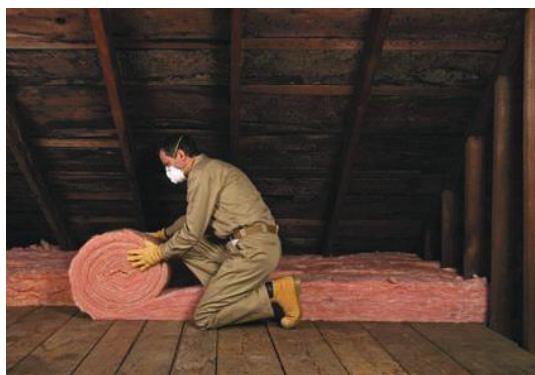
Figure 23.4b Laying lagging in a house loft
